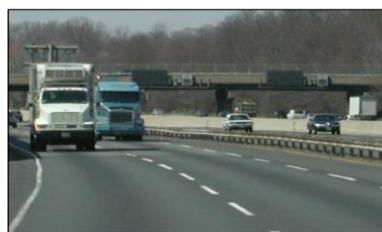
(b) Dual-dual roadway (New Jersey)
