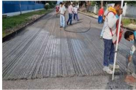
(b) Applying bonding agent
