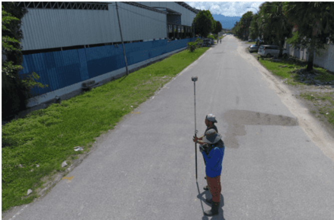
(a) Survey before milling
