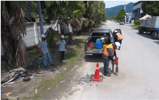
(c) Coring for field testing
