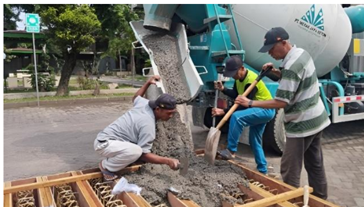
Fig. 2 Casting process of the reinforced concrete beam specimens
