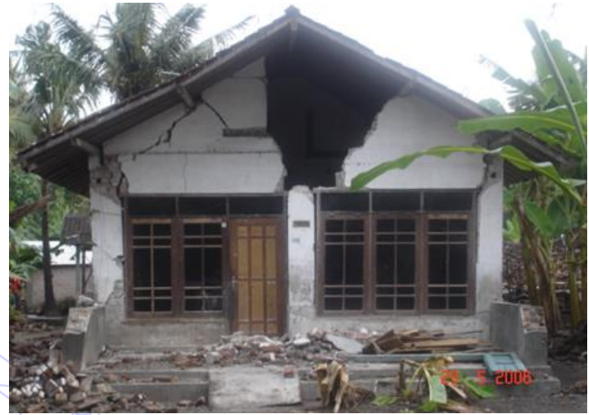
(b) Un-reinforced non-engineered house (Bantul)
