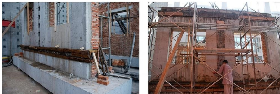
Fig. 4 Pouring of post-cast strips in walls
