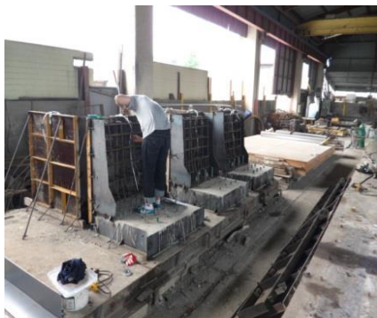
(c) Installation of cast and placement in the barrier
