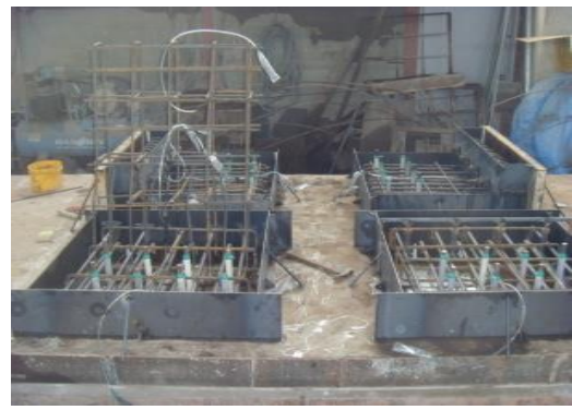
(b) Installation of cast and placement of concrete in the deck
