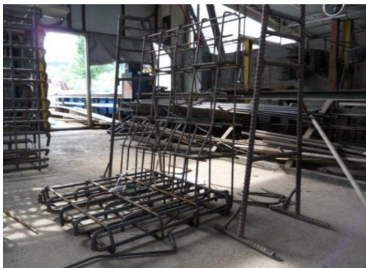
(a) Installation of bar
